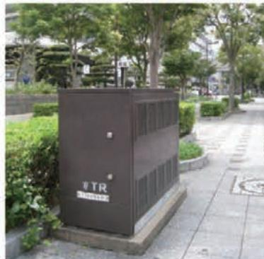
変圧器塔 Pad-mounted transformer
