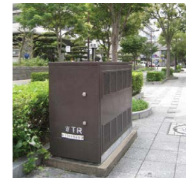
変圧器塔 Pad-mounted transformer
