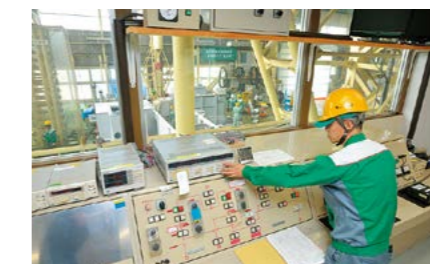
大形変圧器検査場 A facility for inspecting large transformers
