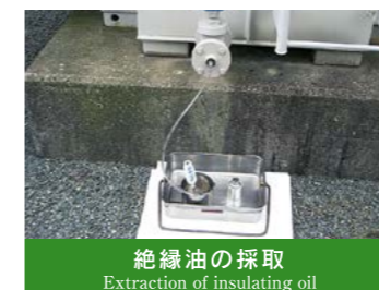
絶縁油の採取 Extraction of insulating oil
