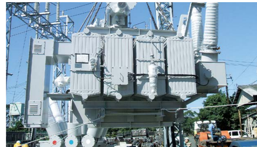
据付工事 Installation in progress
