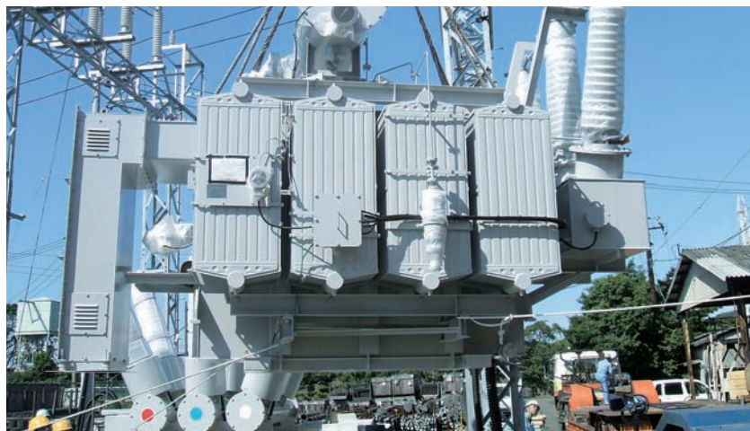
据付工事 Installation in progress
