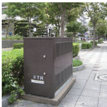
変圧器塔 Pad-mounted transformer
