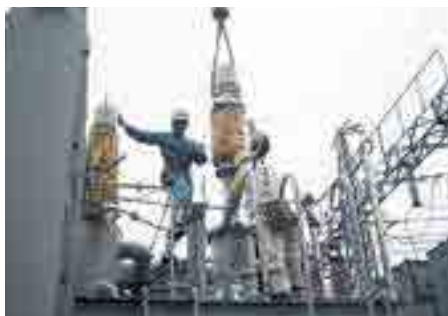
高圧ブッシング取付工事 High-pressure bushing installation work
