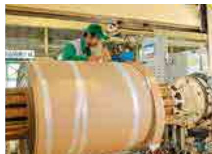
大形変圧器巻線工程 Large transformer coil winding process
