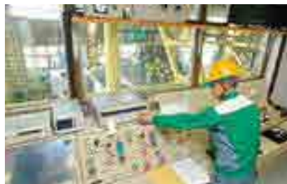
大形変圧器検査場 A facility for inspecting large transformers
