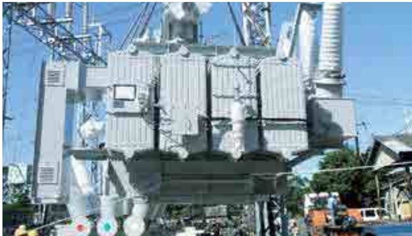
据付工事 Installation in progress
